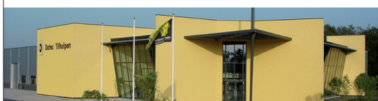
3800 m 2 / 40.000 ft 2 Facility
